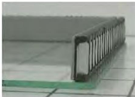
Ensure that spacer is applied 90° to the glass surface.
